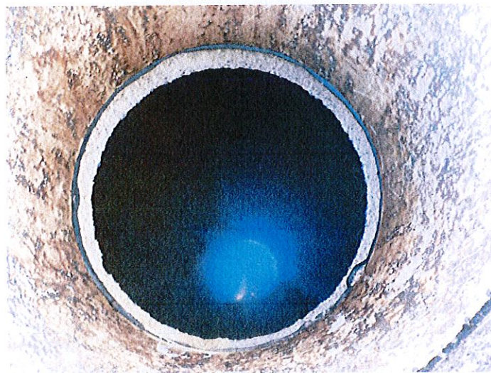
inside of the 2nd tank
