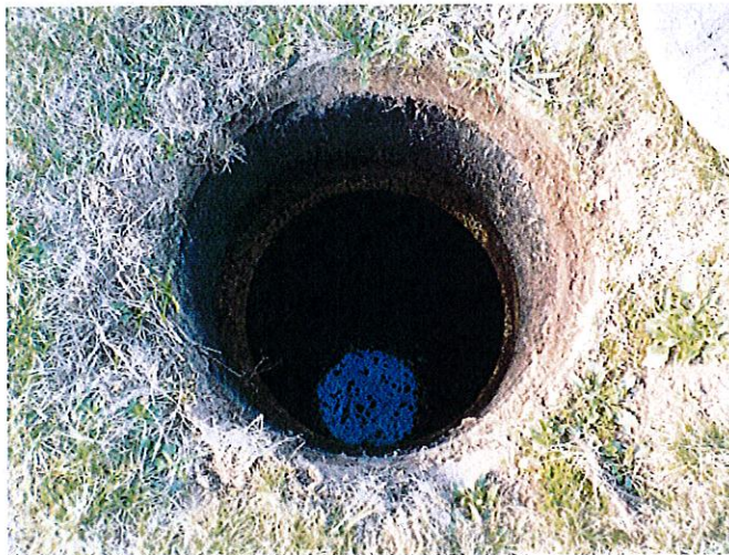
Inside the 1 st septic tank
