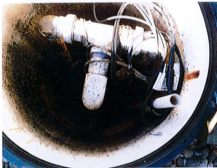
Inside of the dosing chamber
