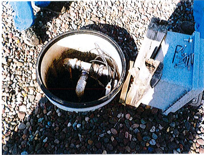
Dosing chamber for the nibbler
