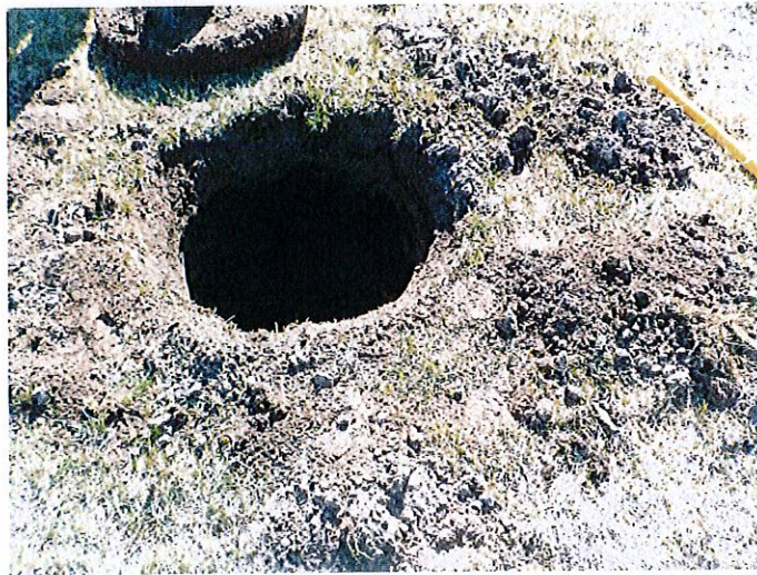
2 nd 1500 gallon tank
