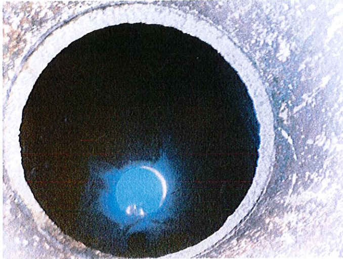
Inside the 1 st tank
