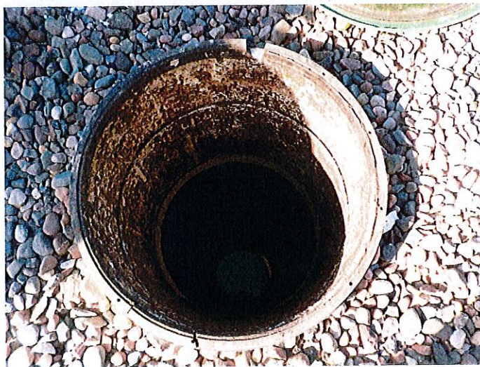
Inside the 1 st 1500 gallon septic tank
