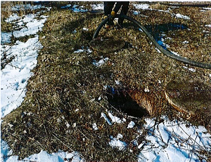
2 nd chamber of the 2 nd 6000 gallon tank
