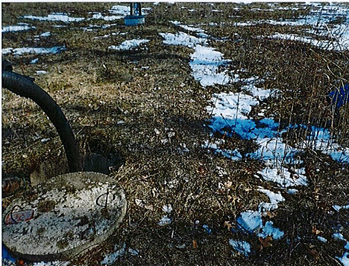
2 nd 6000 gallon split tank
