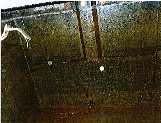
Center wall of the 2 nd 6000 gallon tank
