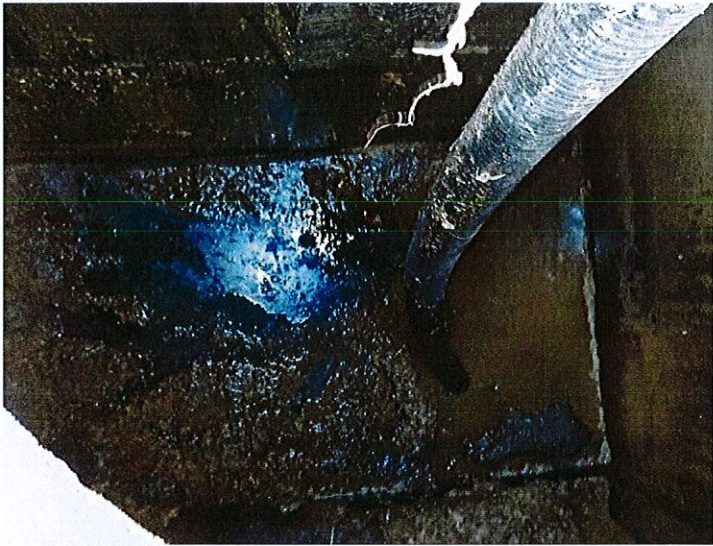
Floor of the 1 st 6000 gallon tank
