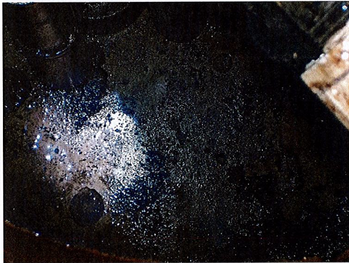
Floor of pump tank
