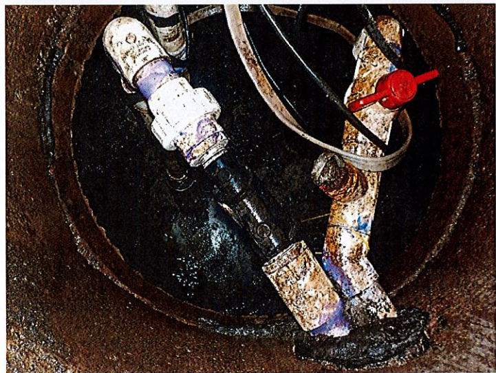
Floor of pump tank
