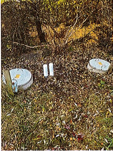
Covers replaced on both the filter and the pump tank
