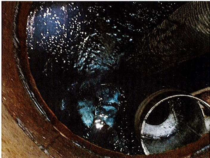
Inside filter tank
